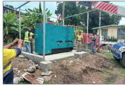
Photo showing the Ground work and the installation of the Twenty (20) Horse power Generator at 6MPC.
