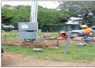
Photo showing the Ground work and the installation of the Twenty (20) Horse power Generator at 6MPC.
